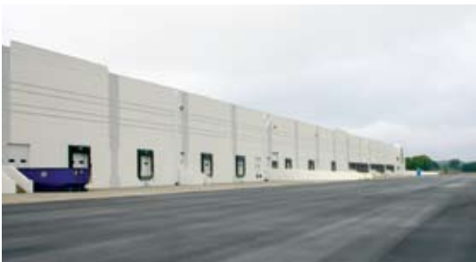
Rear Loading Area
